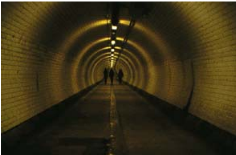
Fig. 2 Woolwich Foot Tunnel, London
